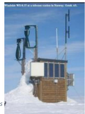
Figure 20 - Example of a twisted vertical axis wind turbine.
